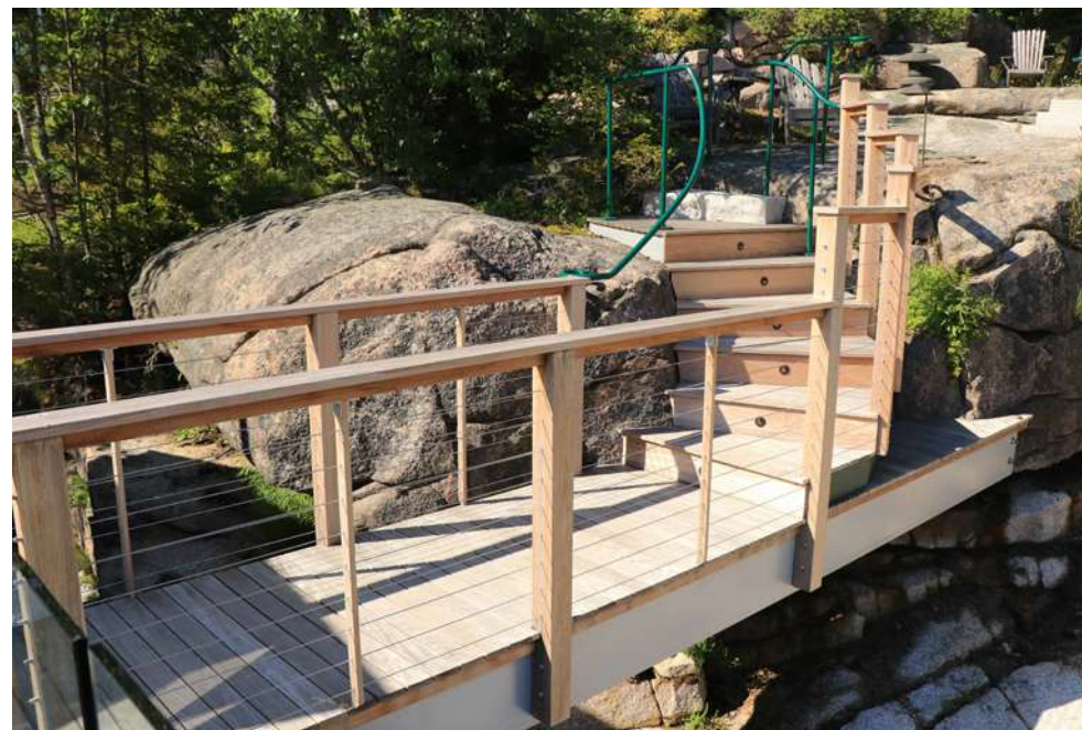
Ipe bridge and iron railings. Steps scribed to ledge.
