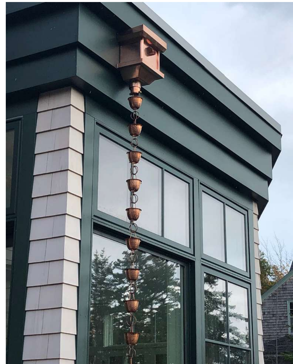
Scupper and rain chain to accommodate green roof irrigation overflow.
