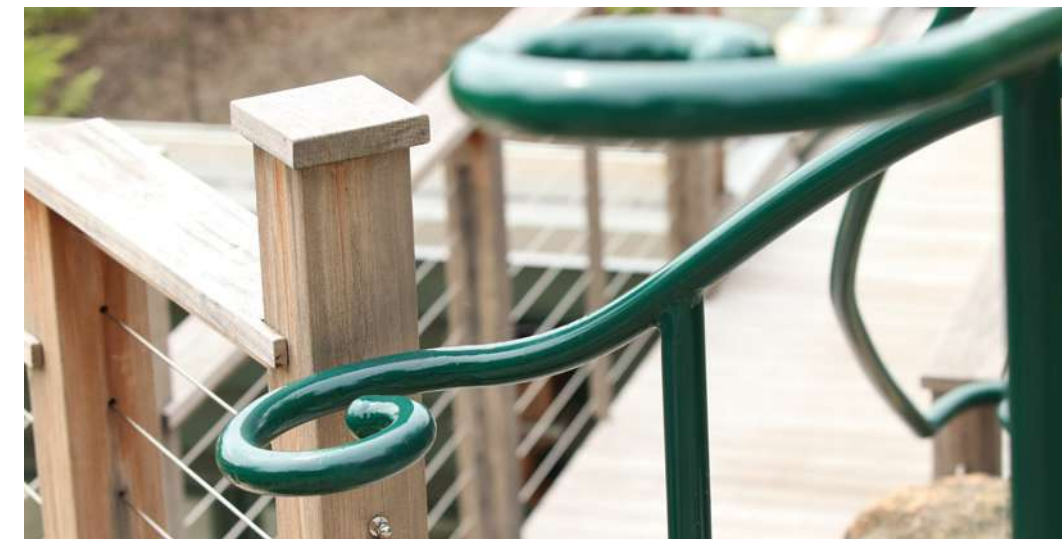
Iron railing meets wood railing – all railings meet code requirements.
